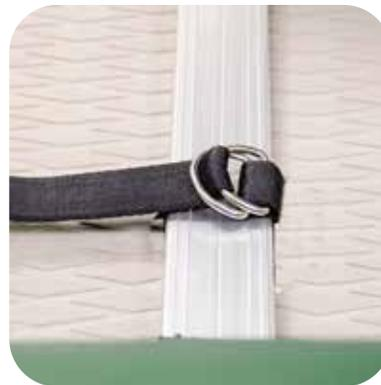
Pull strap tight. Continue securing bar with remaining straps. Check that all are tight.
